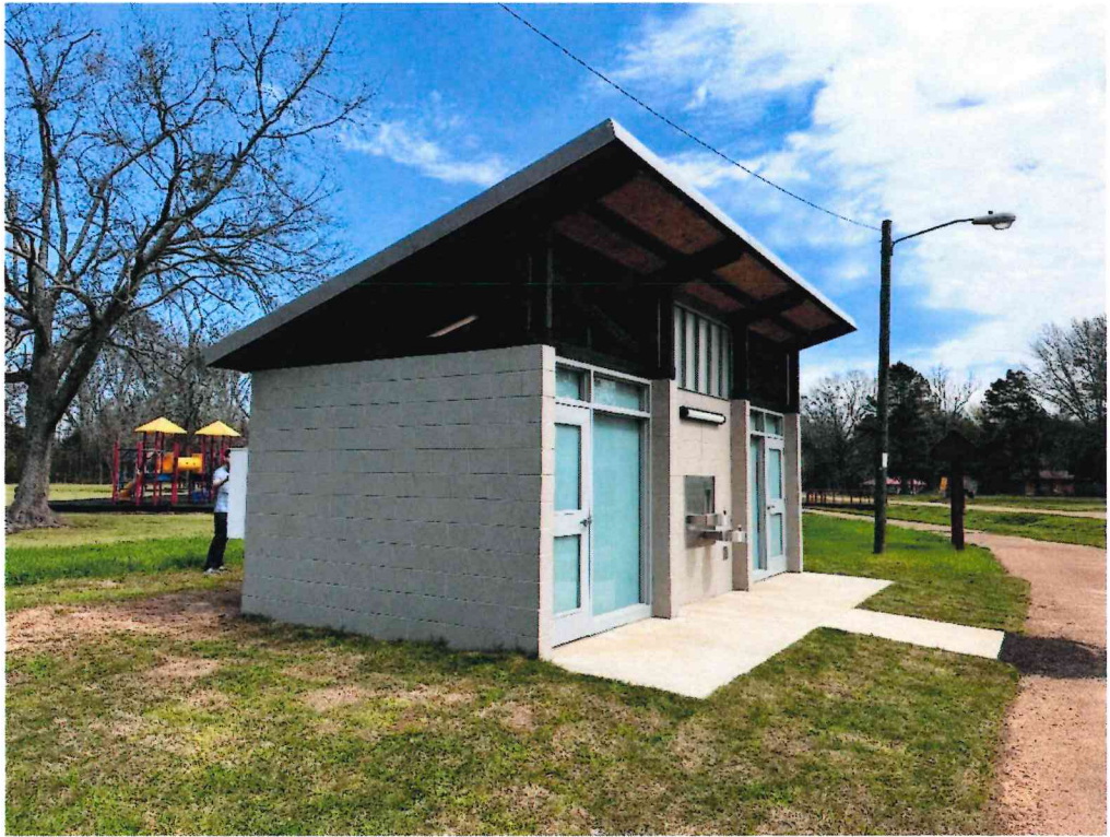
Figure 1 - Estes and Banks nearly complete pending minor corrections.
