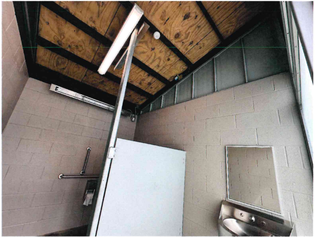
Figure 6 - Estes and Banks nearly complete pending minor corrections.
