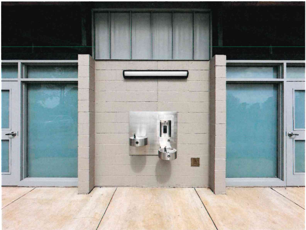
Figure 8 - Estes and Banks nearly complete pending minor corrections.
