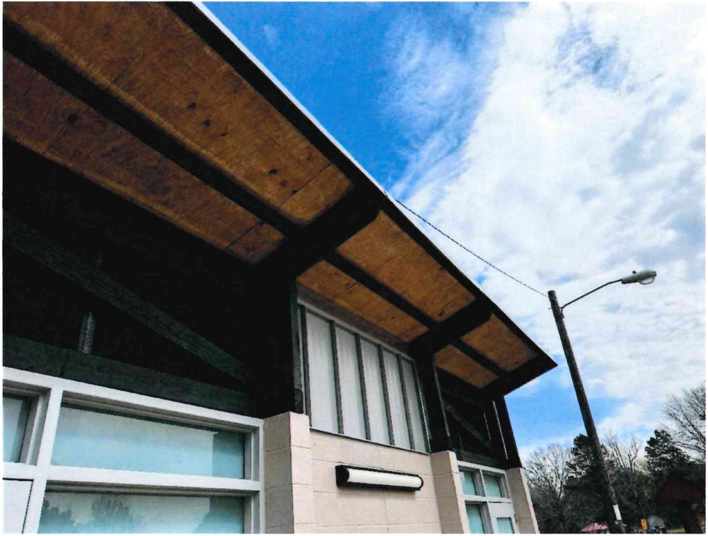
Figure 3 - Estes and Banks nearly complete pending minor corrections.
