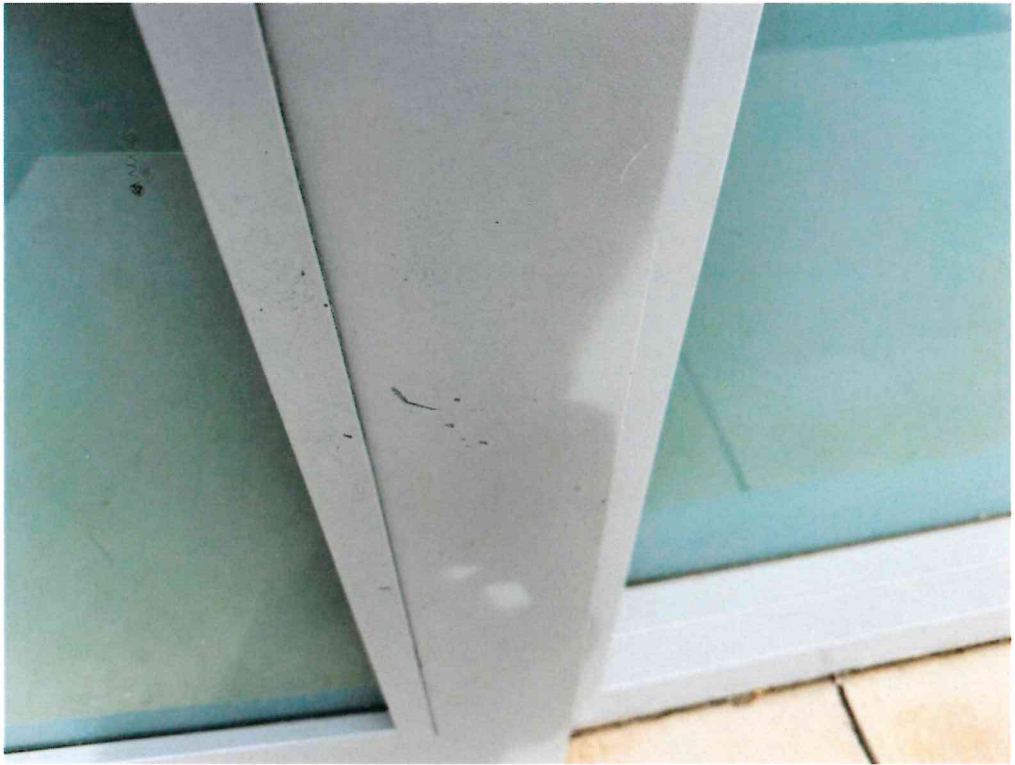
Figure 4 – Touch up paint on frames at all locations.
