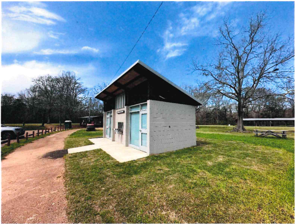
Figure 9 – Estes and Banks nearly complete pending minor corrections.
