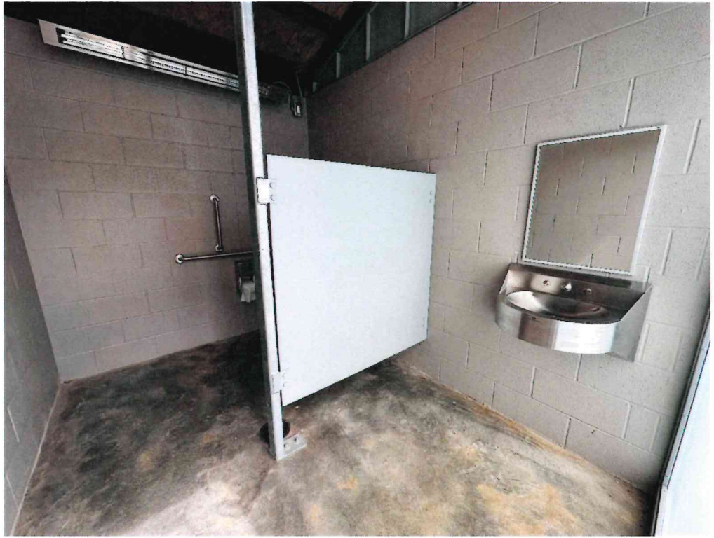
Figure 5 - Estes and Banks nearly complete pending minor corrections.
